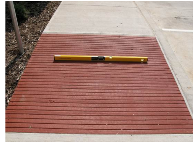
East accessible ramp slope 2.6%
