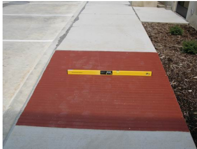
West accessible ramp slope slope 2.6%
