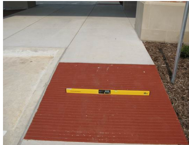
East accessible ramp slope 2.5%
