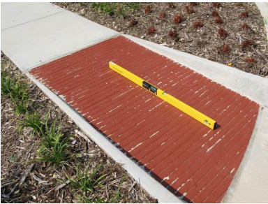
Ramp east of front entry 9% Slope
