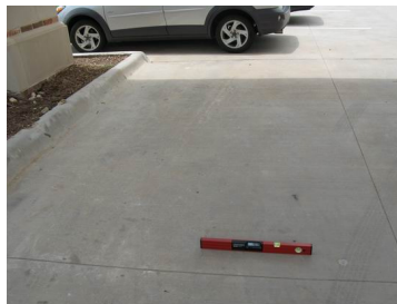
Passenger Loading Zone Slope 2.6%
