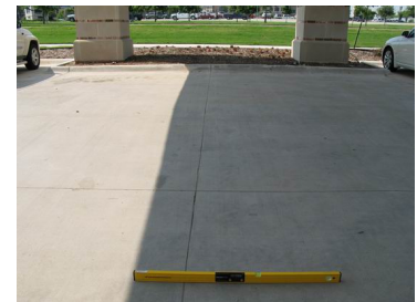
No Access Aisle from Passenger Loading
