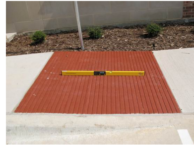
Ramp to public sidewalk 9% Slope
