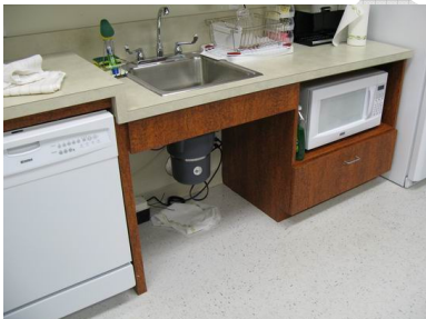
Garbage disposal in Lounge is 6 ½" from the front of the cabinet.
