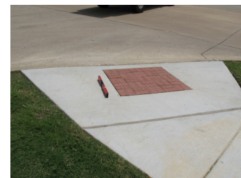
Curb ramp at east sidewalk.
